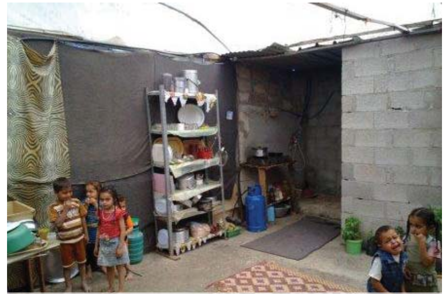
Room with Structural Damage | UUSC
