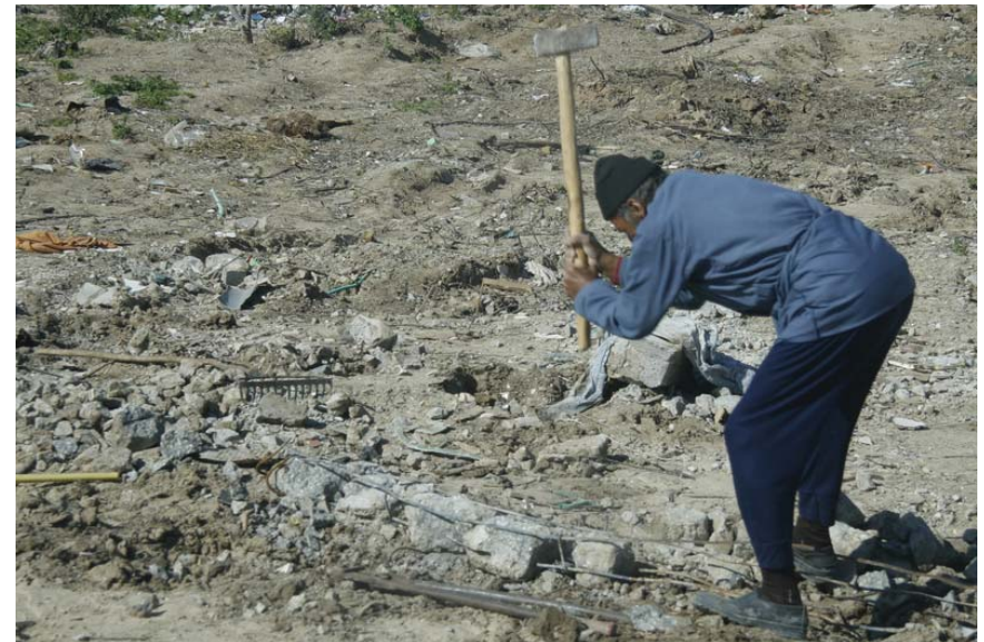
Man straightening steel rebar from used concrete | Gloucester2Gaza
