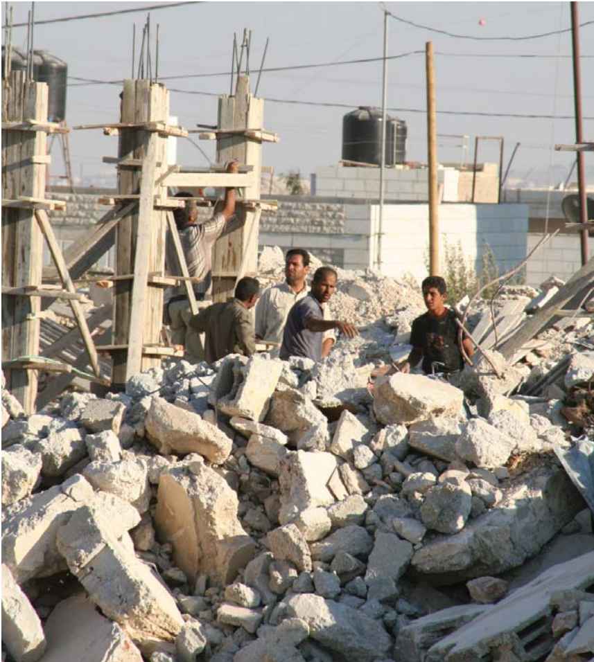
Building in the middle of debris and rubble | Michael Loadenthal flickr.com/photos/michaelimage
